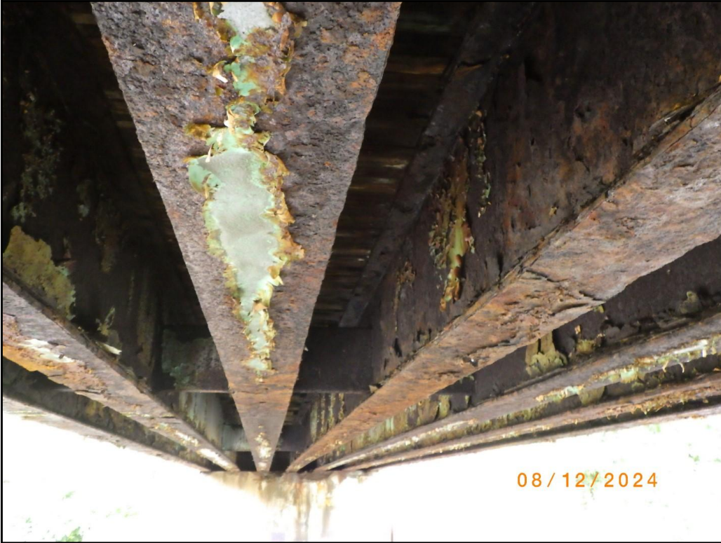
Special Emphasis Detail- Diaphragm Welds.JPG
