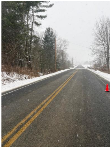
Photograph 3: View of subject bridge from the East.
