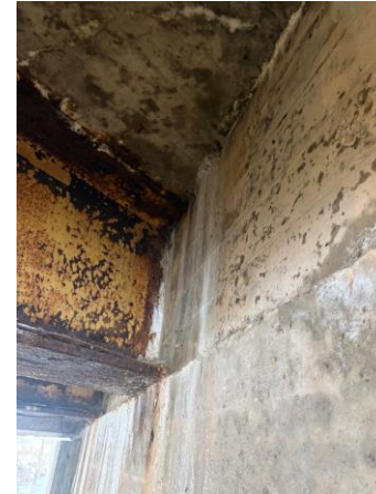
Photograph 2: View of back wall of subject bridge.
