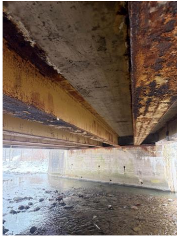
Photograph 1: View of yellow paint on bridge girders of subject bridge.
