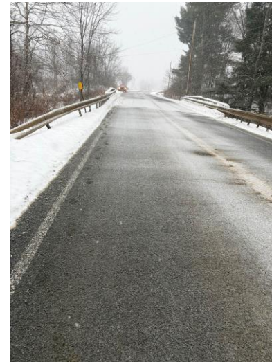
Photograph 4: View of subject bridge from the West.
