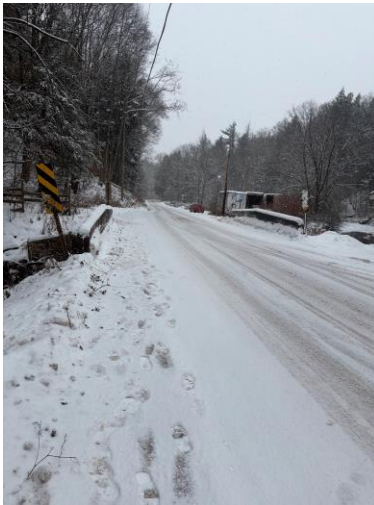
Photograph 3: View of subject bridge from the Northeast.
