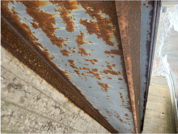
Photograph 1: View of light gray paint on bridge girders of subject bridge.
