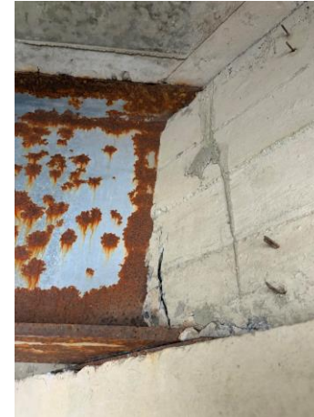
Photograph 2: View of back wall of subject bridge.
